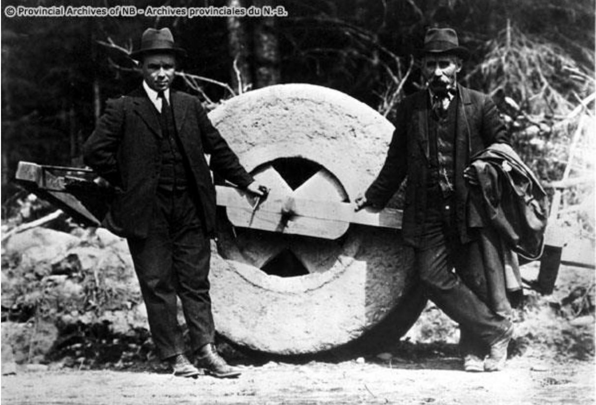
Two men standing in front of stone roller while doing road work in York County.
